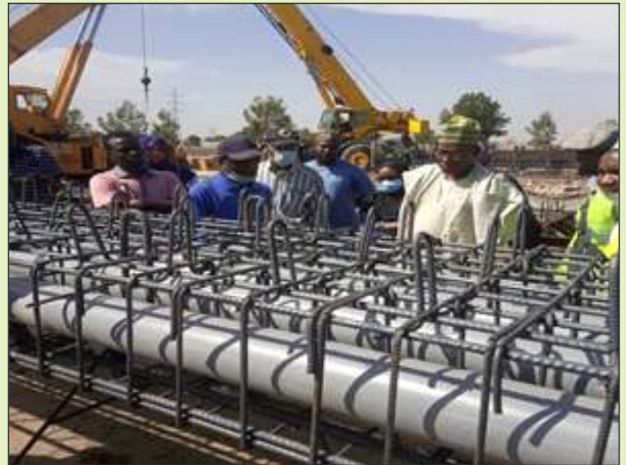
Physical Inspection of Reinforcement at one of the Projects Site.
